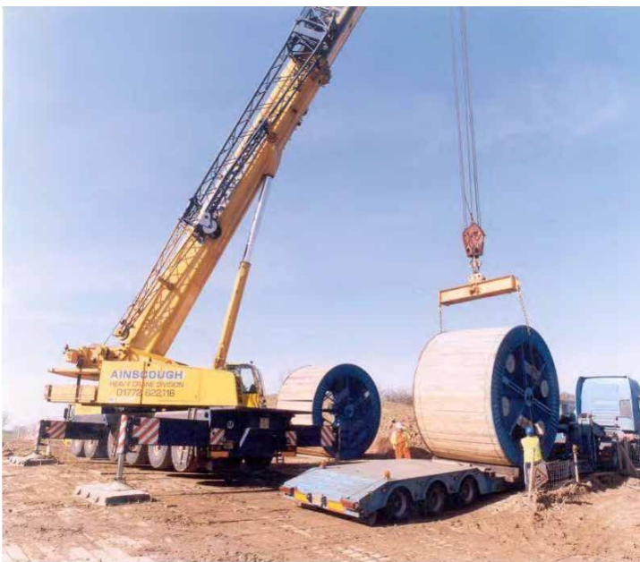
Figure 40 – Offloading cable drums
