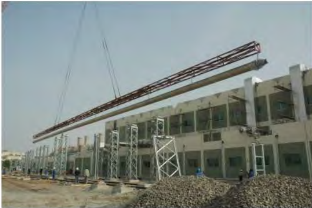
Figure 62 – GIL segment being lifted into position
