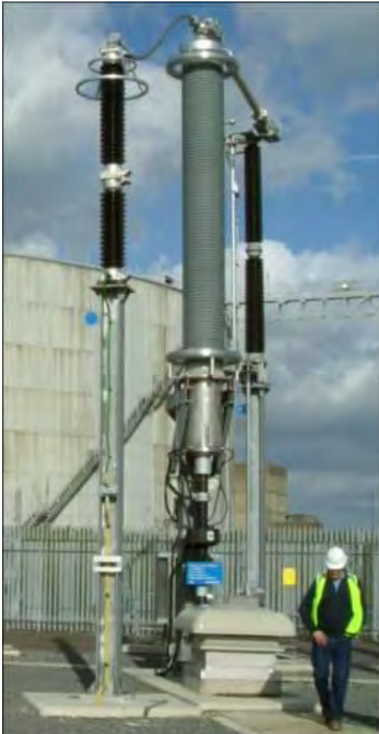
Figure 21 – 400kV cable outdoor sealing end (ODSE) termination
