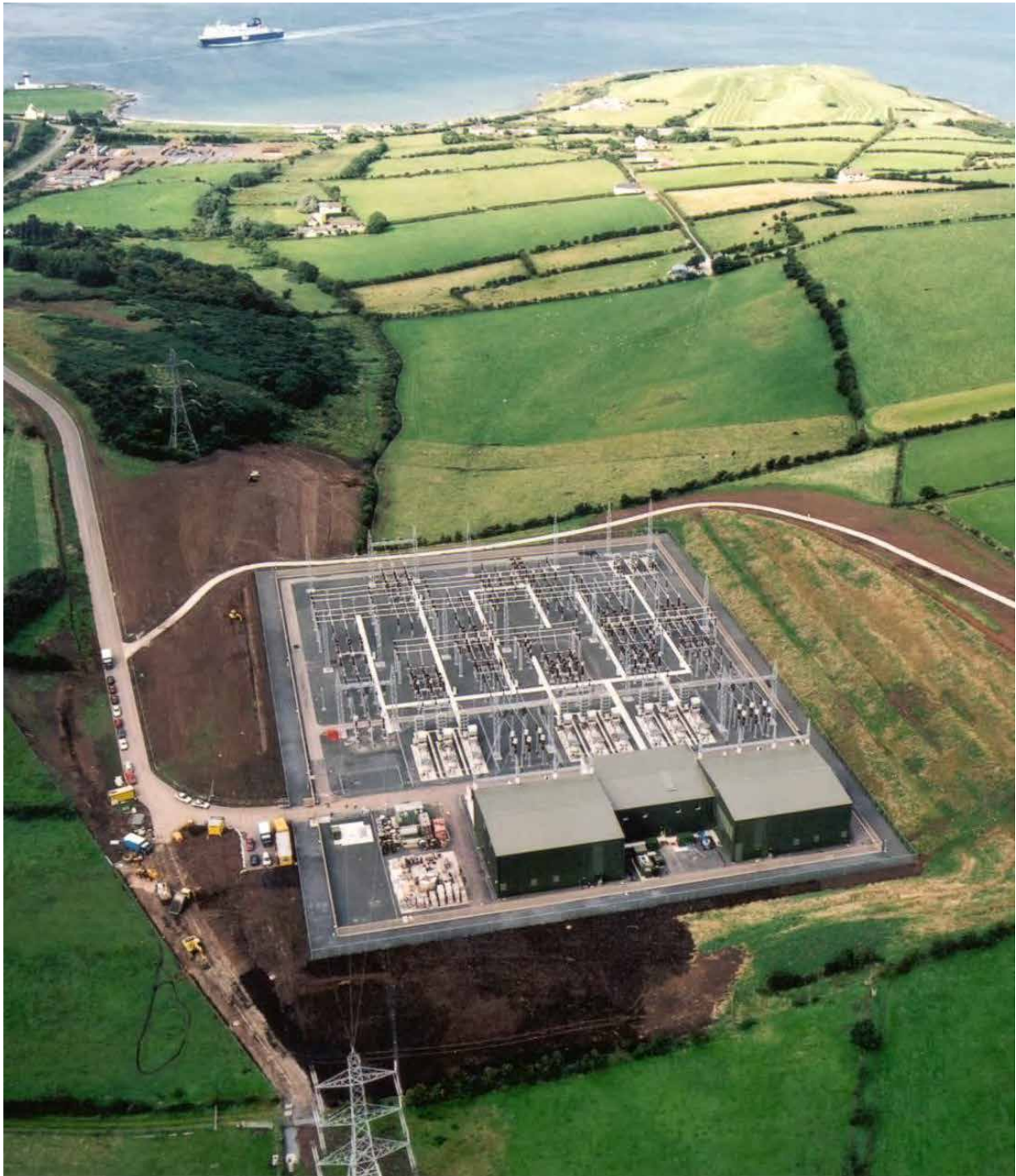
Figure 5 – Ballycronan More 500MW CSC converter station
