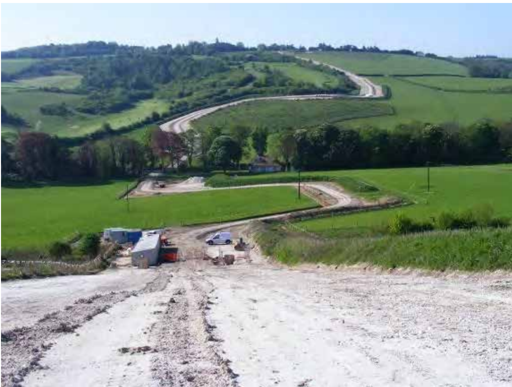
Figure 35 – 400kV cable swathe at the Goring Gap
