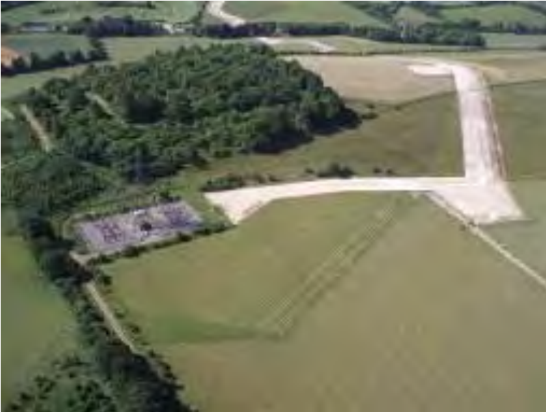
Figure 24 – Moulsoford Down 400kV SEC near Goring
