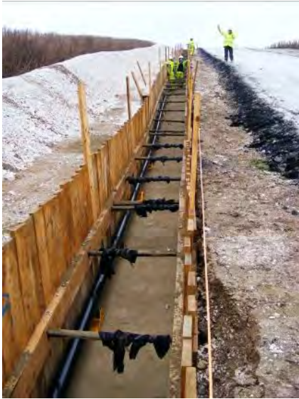
Figure 41 – Cable installation in an open cut trench
