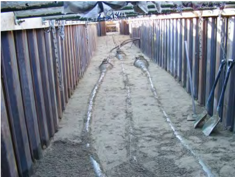
Figure 19 – EHV joint bay containing three Joints
