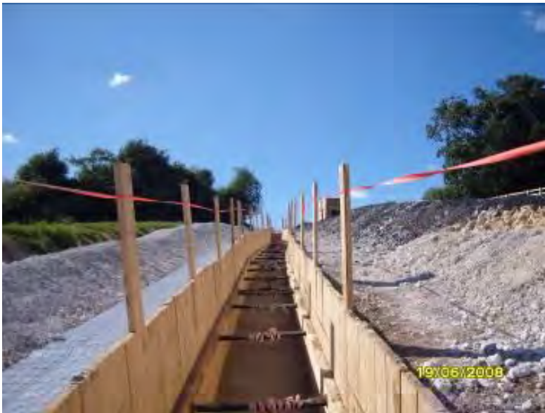
Figure 37 – A close-timbered cable trench
