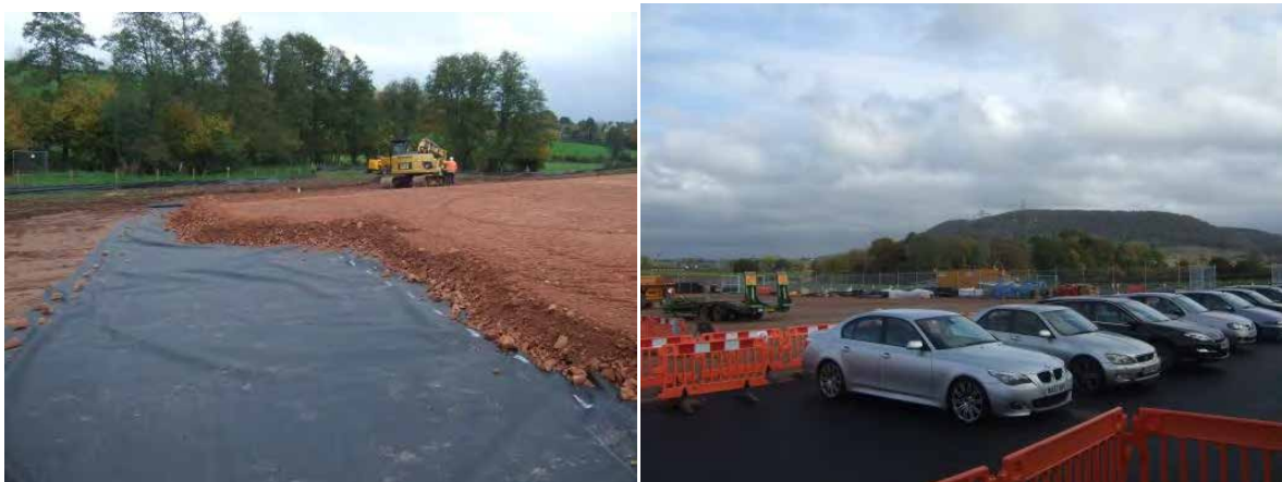
Figure 28 – Site storage/laydown area and site administration
