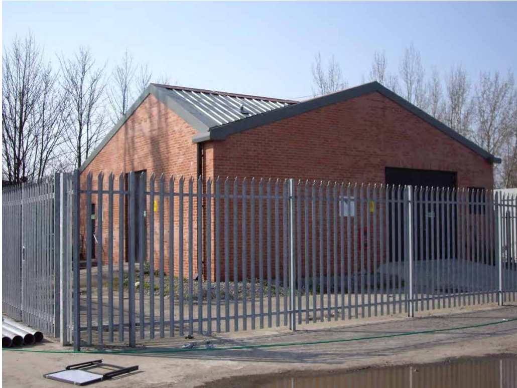
Figure 72 – Completed shaft head-house, within a secure compound
