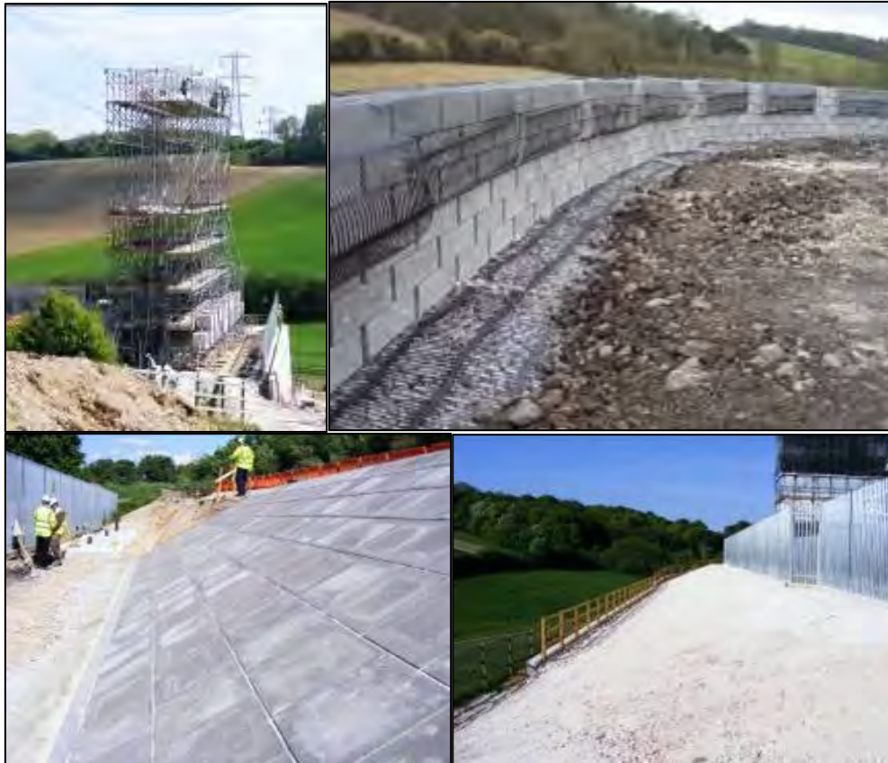
Figure 30 – Retaining walls and earthworks (enabling works)
